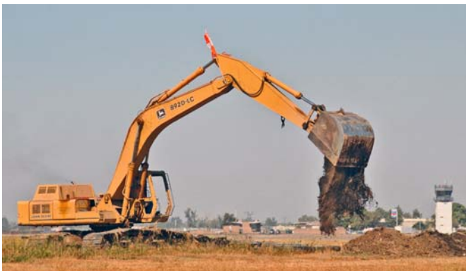
Pipeline Irrigation and drainage canal project under construction.
